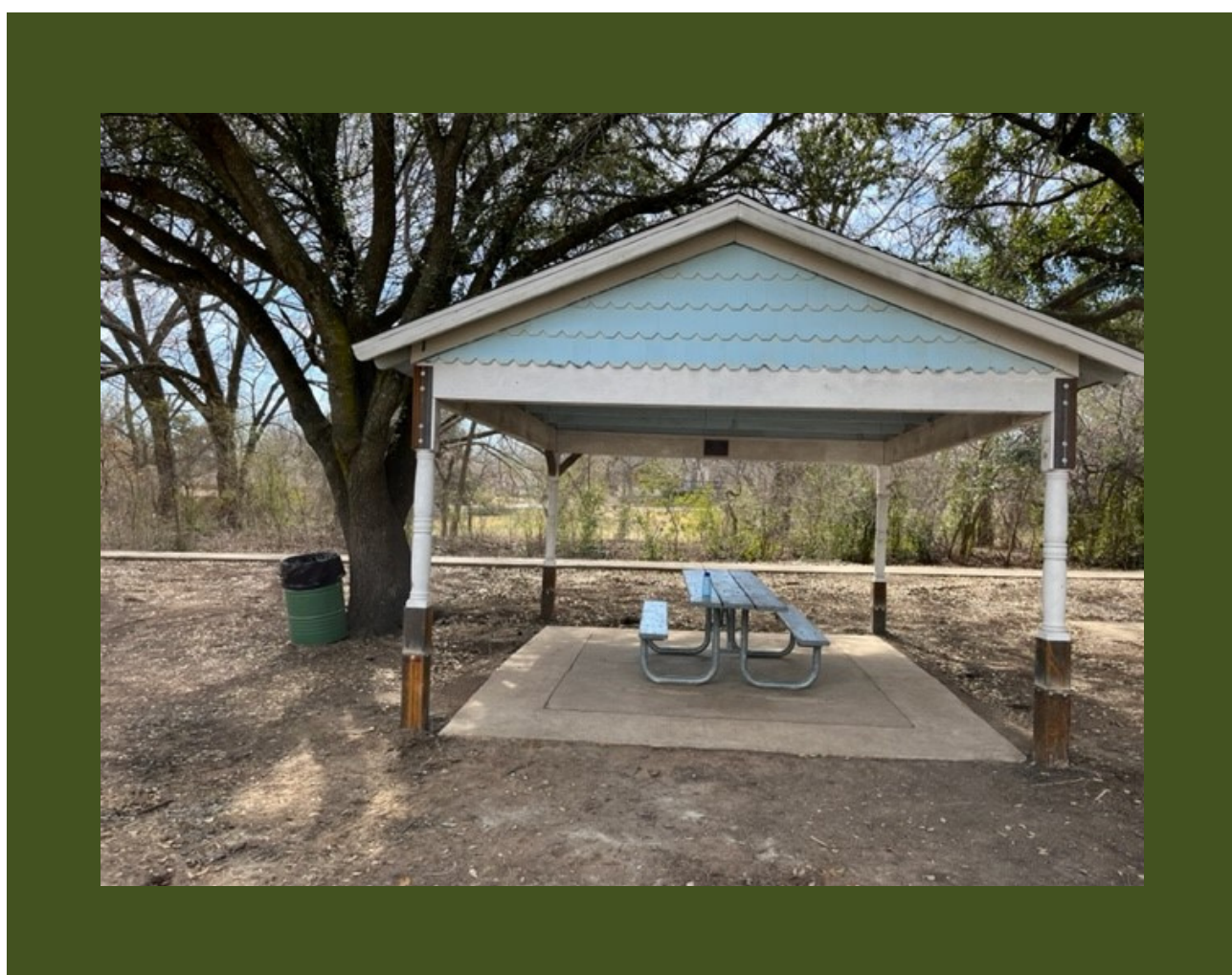
PAVILION REPAIR AT LOFLANC PARK
